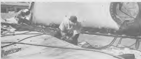
A WORKMAN, above, trims tank plates prior to installation on the bunker station's building site. Applying a weld, left, to one of the storage tank's bottom seams is an employee of Curaçao Dokmaatschappij, one of the bunker station's two contractors. UN TRAHADOR, arriba, ta trim plachinan di tanki promer cu nan worde instala. Aplicando un weld, robes, na bon di un di e tankinan ta un empleado di Curaçoesche Dokmaatschappij, un di e dos contratistanan di e stacion.
